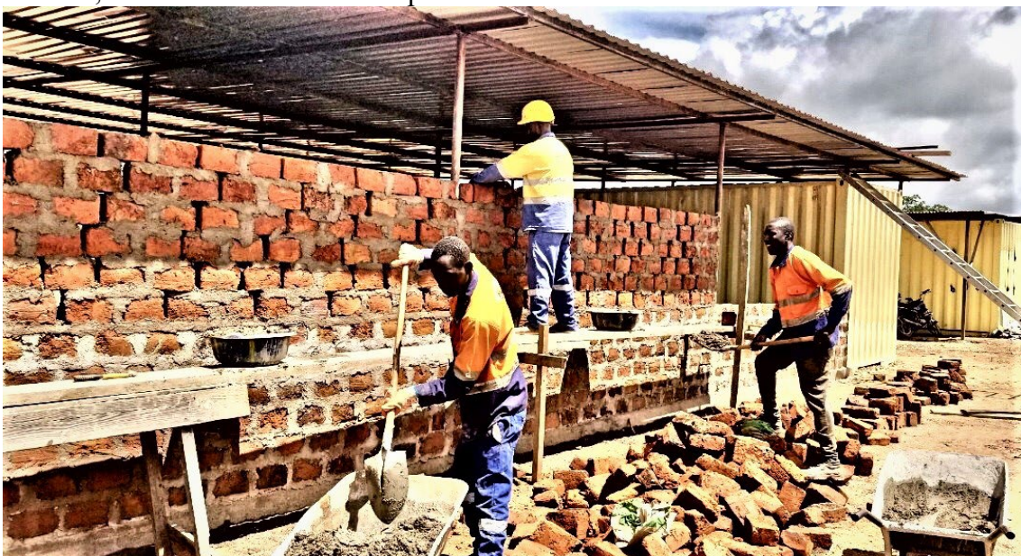
Figure 3.6 New industrial building under construction
