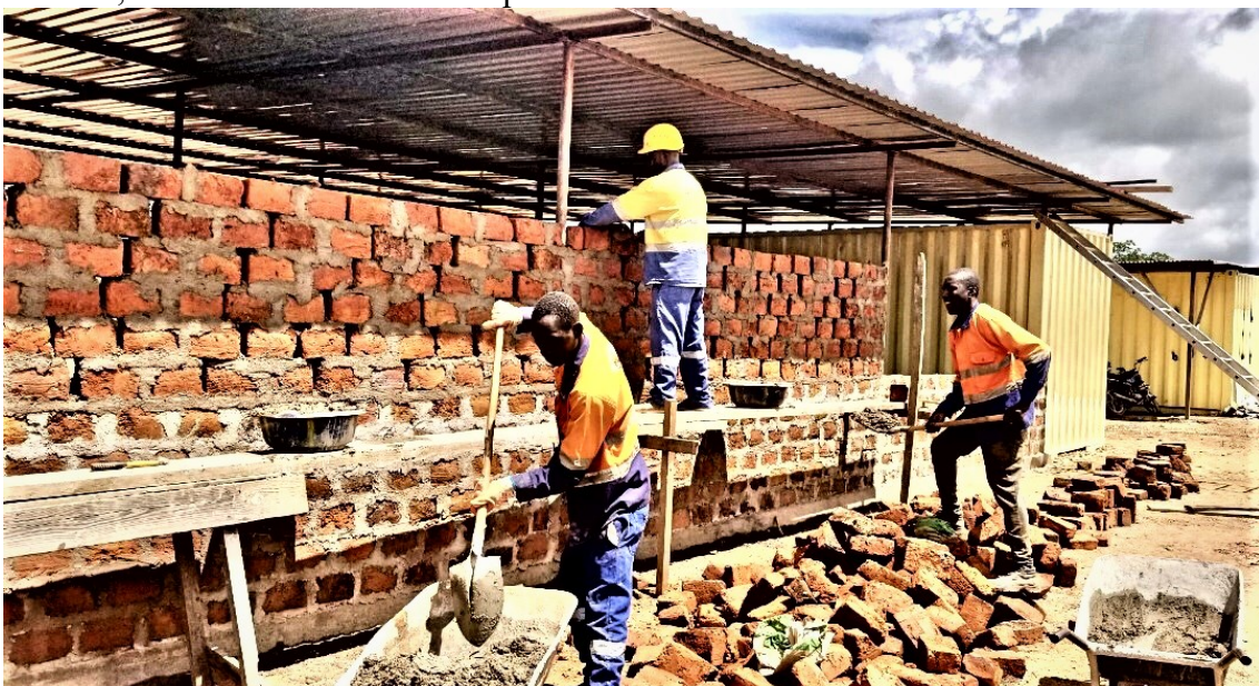
Figure 3.6 New industrial building under construction
