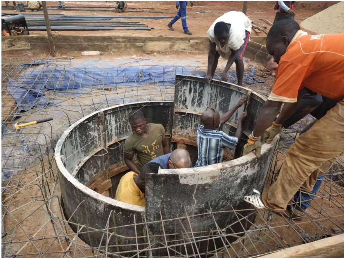
Figure 20 Start of the shaft construction
