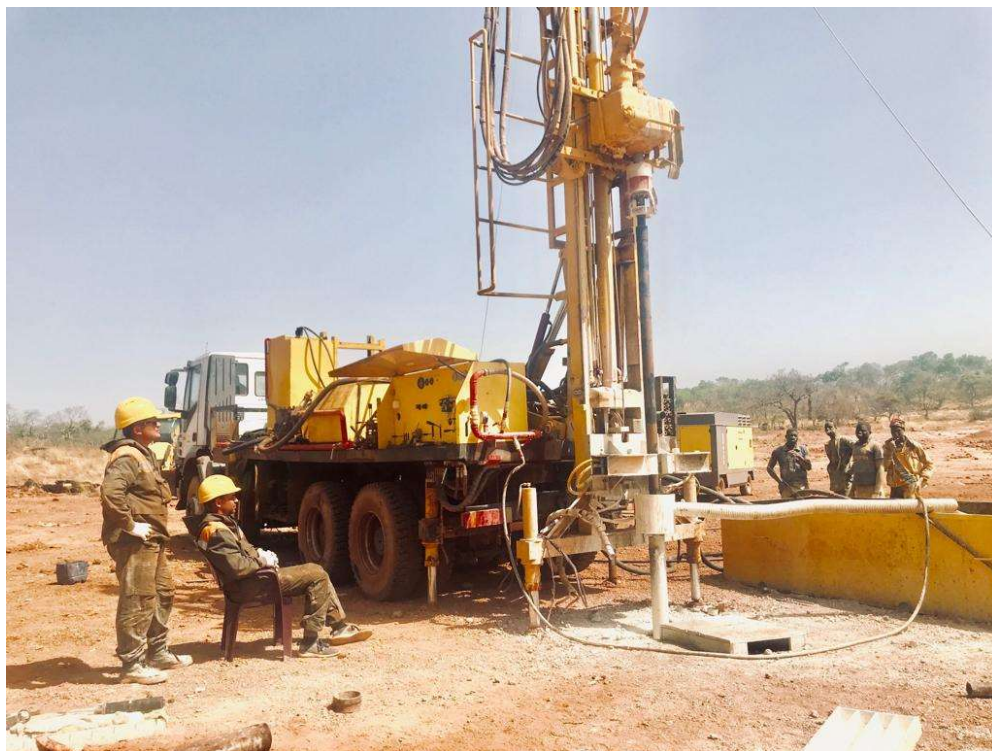
Figure 17 – Gelecs 200 drilling installation during exploration drilling with Boart Longyear equipment
