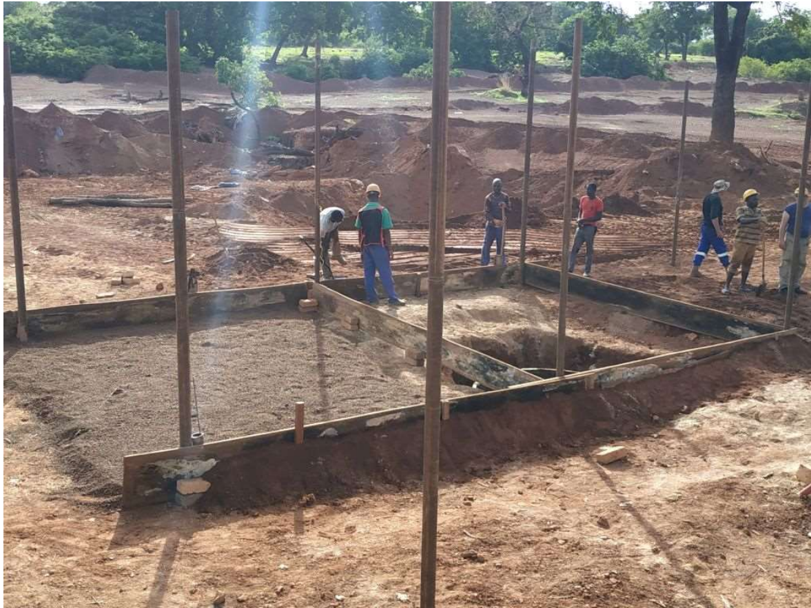
Figure 15 Commencement of the first shaft construction
